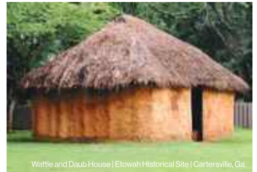
Wattle and Daub House | Etowah Historical Site | Cartersville, Ga.
